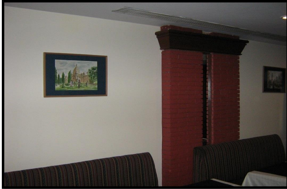
Illustration 31: Existing status of the walls of the Restaurant
